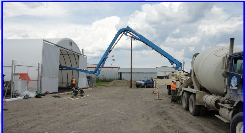
Figure 2 Pumper-Truck pumping concrete for a concrete pad INSIDE an existing structure.
