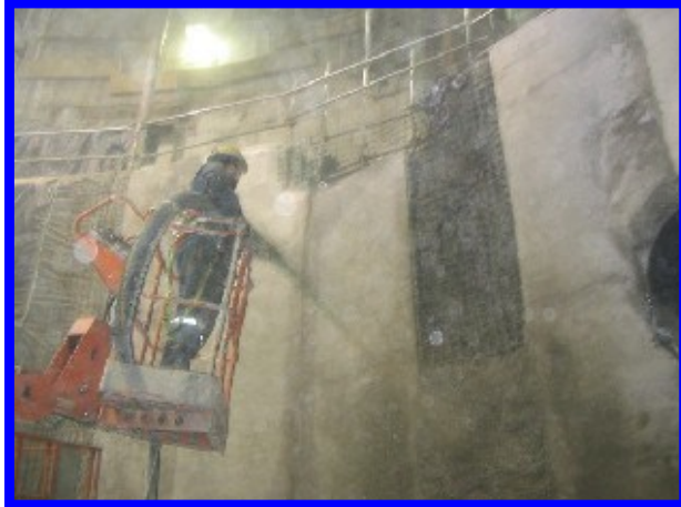
Fig 3 Application of Shot- crete to Basement
