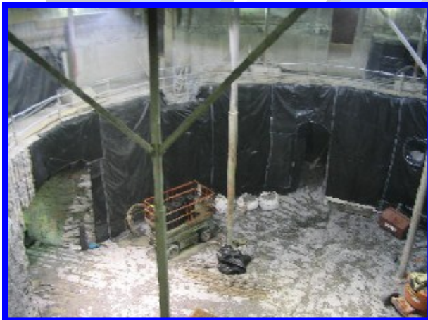
Fig 5 Main Excavation of Basement Levels
