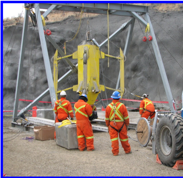
Setting up the Raise Robot® over the Vent Raise
