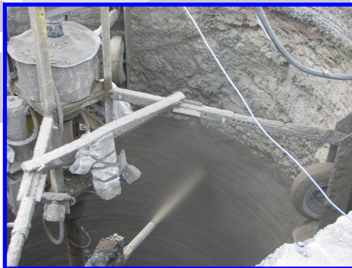
Raise Robot® Completing Top Meter of 3.5 m x 300 m Deep Raise
