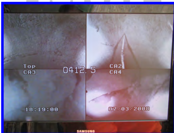
Split Screen Viewing of Shotcrete Application
