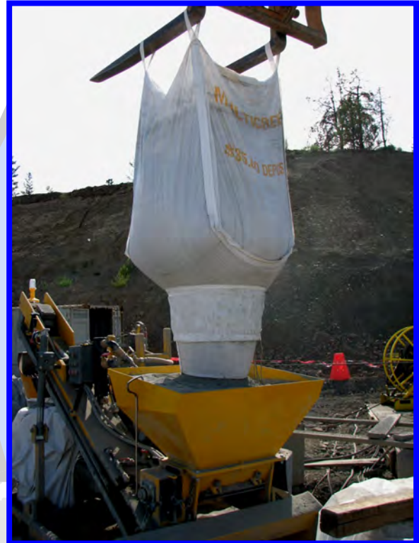
Bulk Bags of Dry Pre-Blended Shotcrete Suspended over Predampener Hopper
