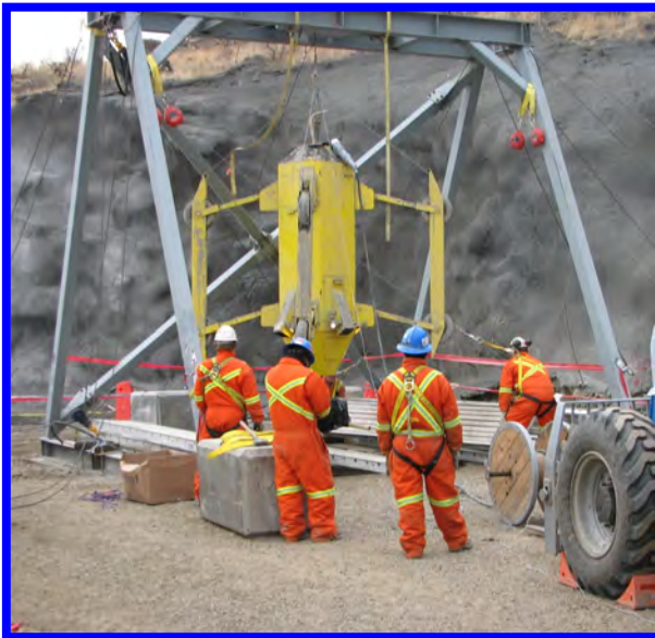
Setting up the Multicrete Raise Robot™ over the Vent Raise
